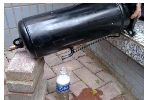
Figure 2: Draining oil from a compressor
